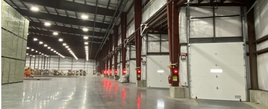
SOUTHERN TIER LOGISTICS BUSINESS PARK
