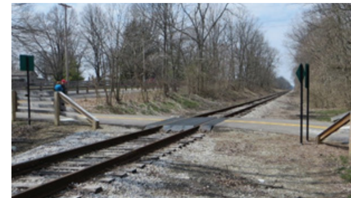
Example rail crossing, adequate sight distance, advance notice of crossing, perpendicular to trail, smooth crossing surface. (Rails-to-Trails Conservancy)
