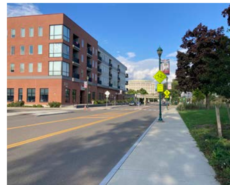
Water Street, City of Elmira with signed shared bikeway with sidewalks.
