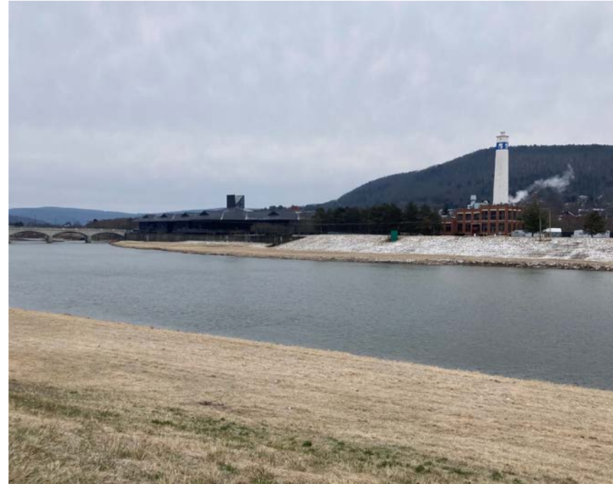
Corning Incorporated Headquarters from path along Hillvue Avenue and the Chemung River.
