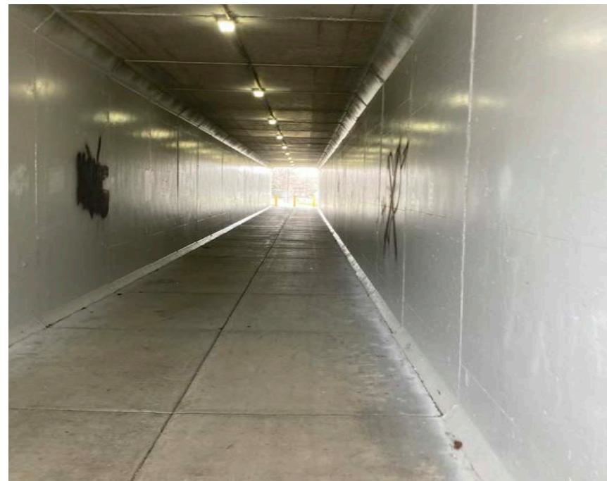
Existing Highway Underpass, opportunity for improved lighting, community art projects.
