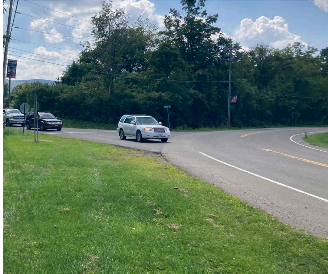
Intersection of Maple Street and Winters Road, location of proposed roadway overcrossing.
