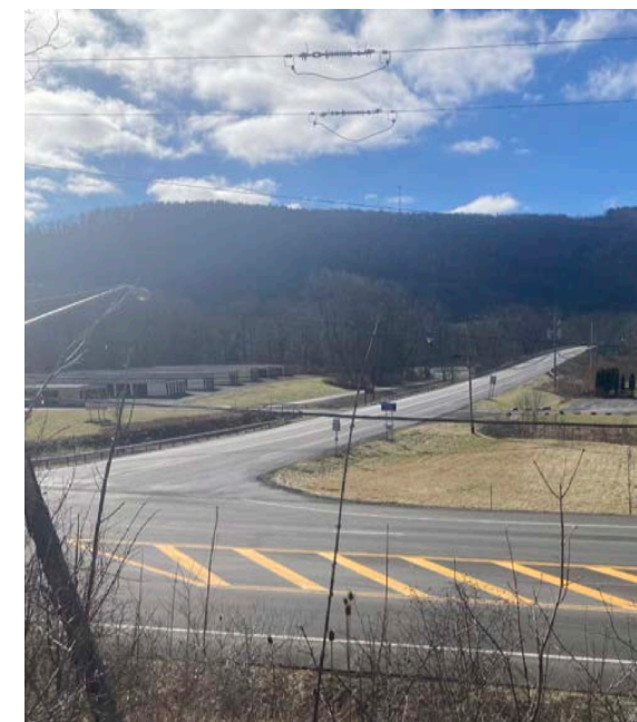
Hendy Creek Road and NYS Route 352 Intersection.
