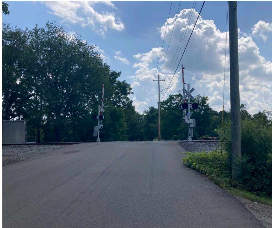
Hammond Street Railroad Crossing.
