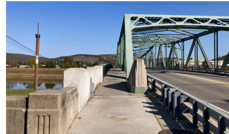
Sidewalk between Bridge Street and Wegmans, Bridge Street bridge looking north.
