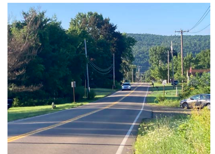
Goff Road looking south from Feeder Canal.
