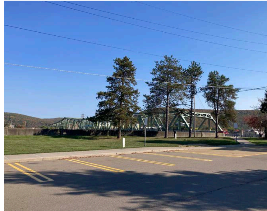
Proposed Trailhead area at Wegmans parking lot near Bridge Street bridge.
